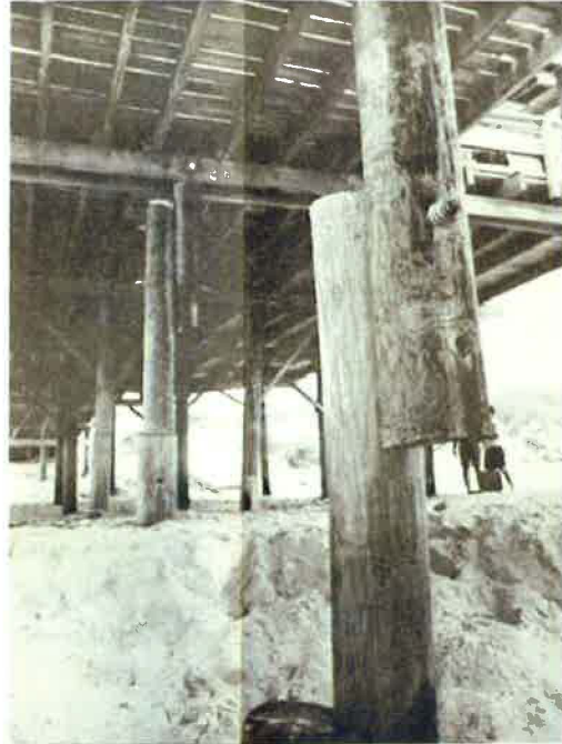
1975 Images of Frisco Pier Pilings Showing Repairs (ACOE)
